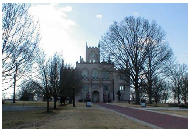
Wartime capitol in Milledgeville. Interior visits have been suspended due to virus restrictions. We believe the building will be open by October.
