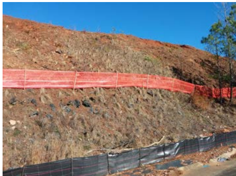
View of the site from Dallas Highway, looking north.
