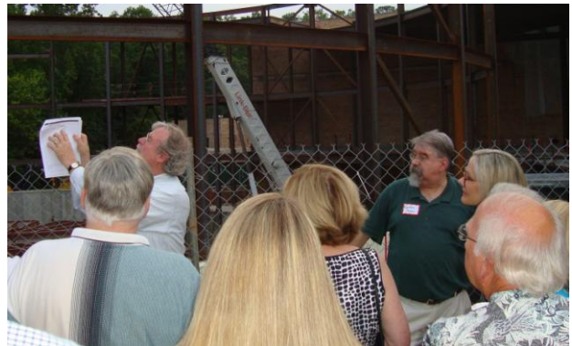
Architect Grant Moseley (left) explains features of the new building. History Center curator Gordon Jones is in dark green shirt at right.
