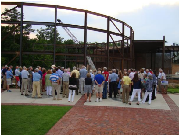
Civil War Round Table members gather at the framework of the new building.
