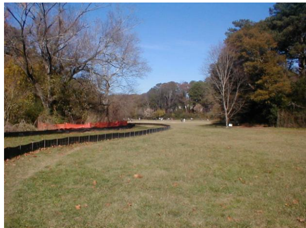
Course of the future bike path is visible to the left, shortly before it turns westward to cross Tanyard Creek, leaving most of the meadow as open space.
